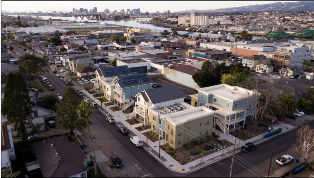
An affordable housing project in Alameda County in Northern California.
