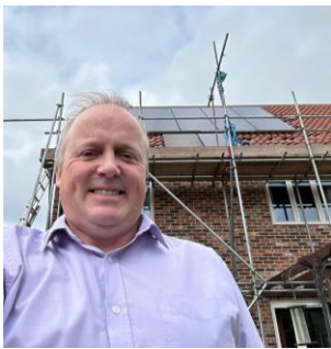
Solar panels being installed on my roof
